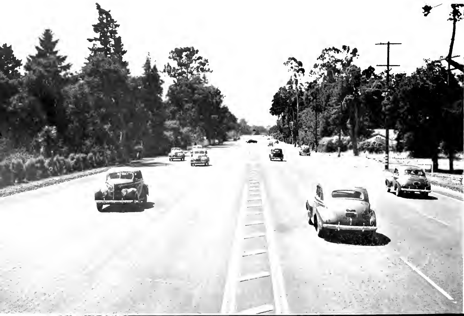
Typical view of widened section of U. S. 101 near Atherton providing a 6-lane divided highway
